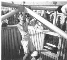
Emergency housing project using standard cardboard tubes, Kobe, Japan Shigeru Ban, architect
