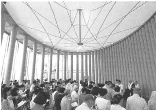
Emergency housing project using standard cardboard tubes, Kobe, Japan Shigeru Ban, architect
